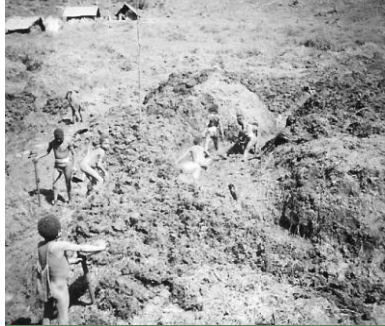
Constructing an Airstrip
